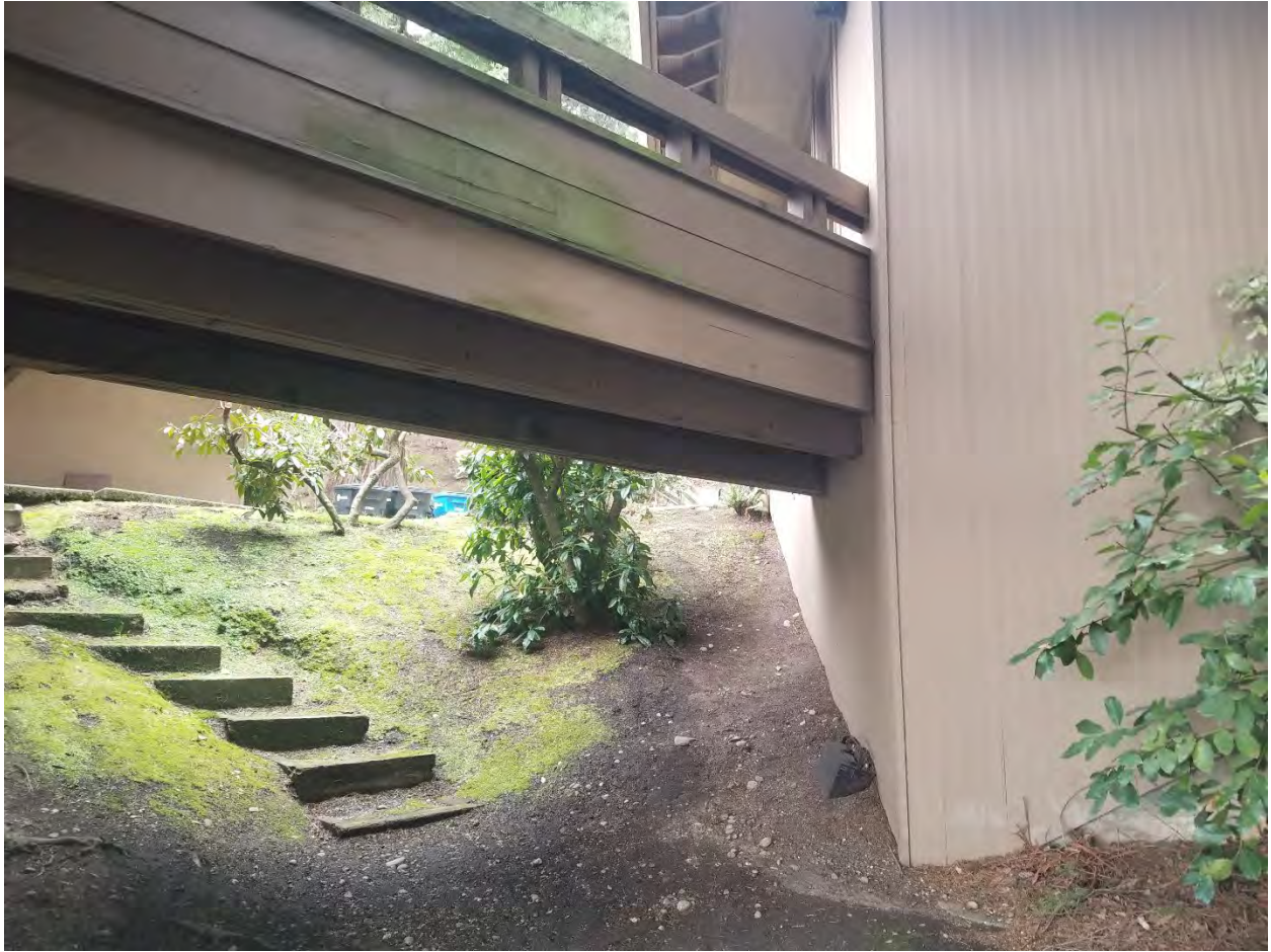
Ground Walkway Under Wood Bridge Between House and Garage
