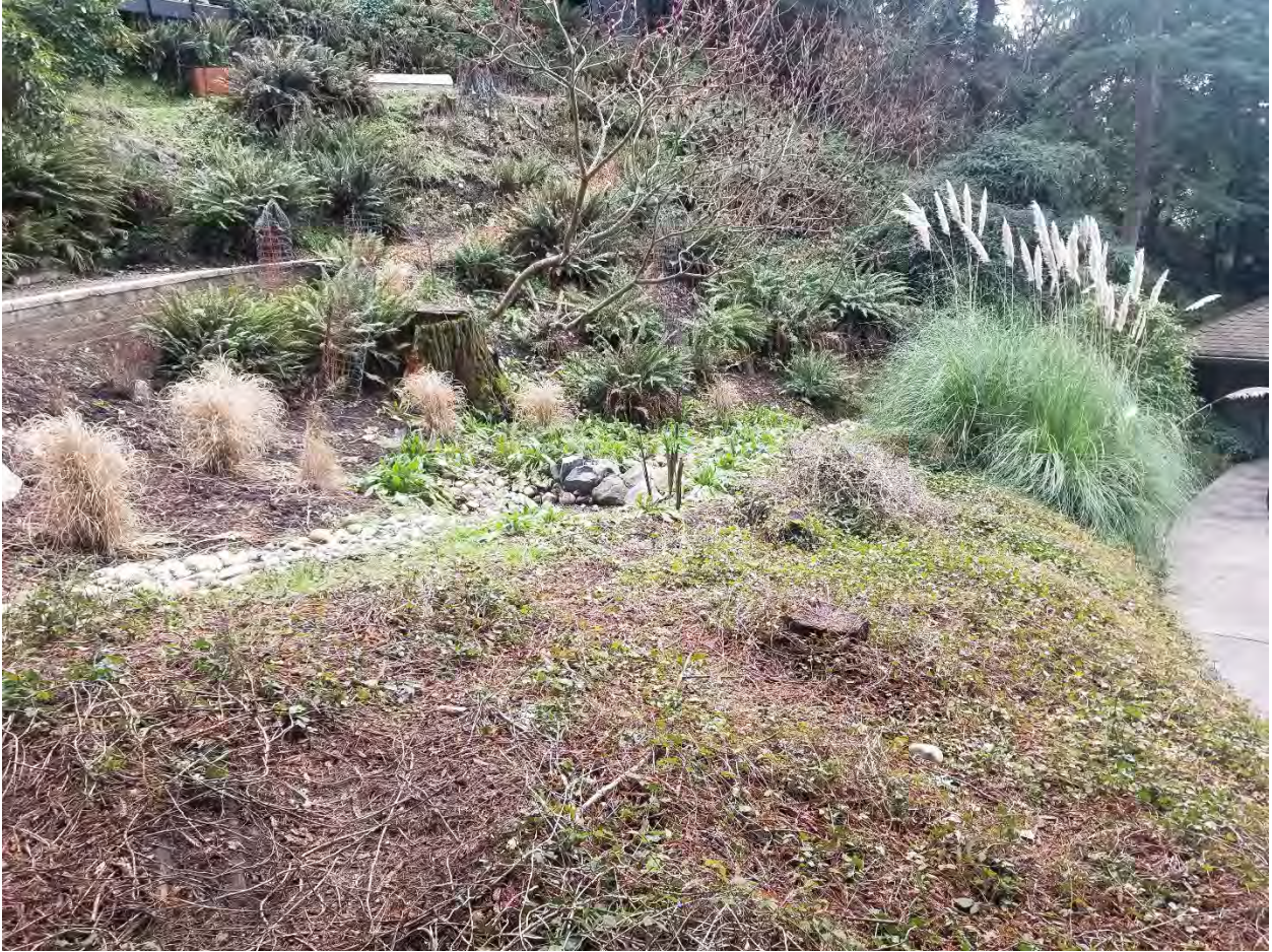
Rock Lined Swale on Neighbors Property Above Driveway
