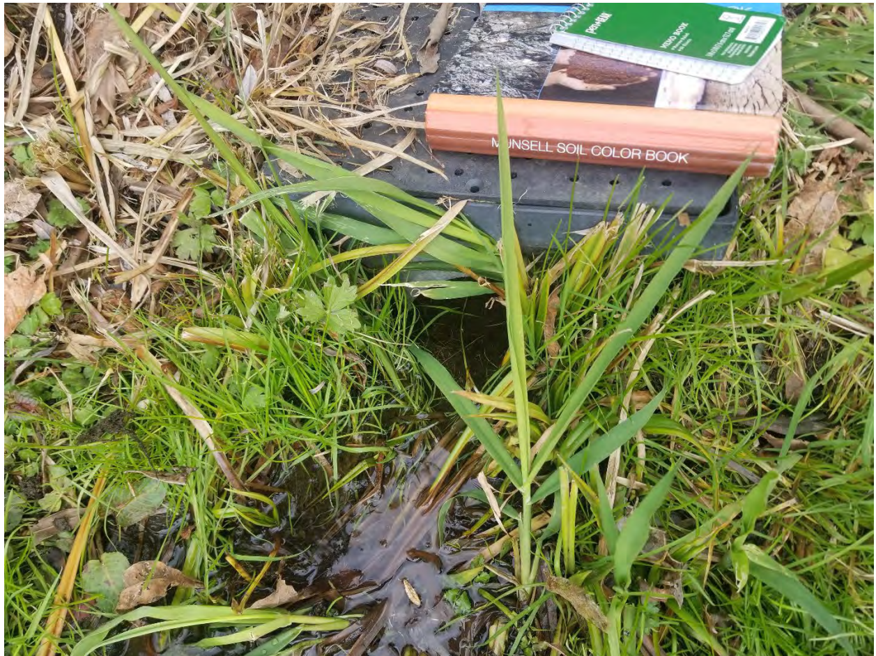
Wetland Pipe Box Outlet
